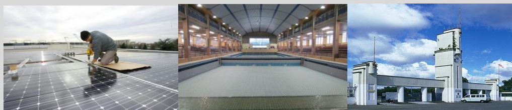
Photo 1 : Installation of the solar panels on the Nakache Swimming pool
